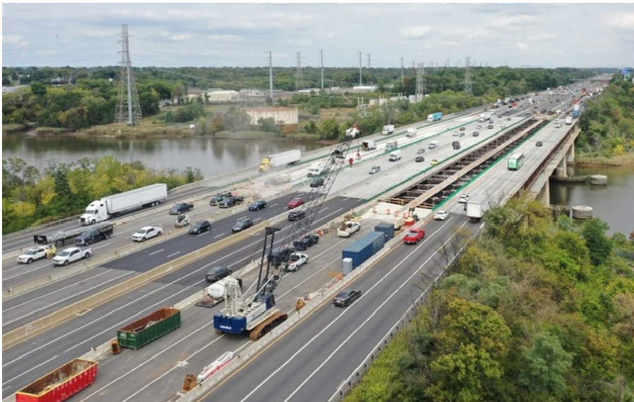
Figure 4: Contract T100.523 Bridge Deck Reconstruction Mileposts 83 to 88
