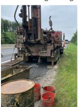
will determine the types of foundations required for the various structural elements (such as bridges, sign structures, ramps) and if the soils are suitable for the roadway to be constructed on. If the soil materials are soft or loose and not suitable to be built directly on, a deep foundation system or other soil improvement techniques will be required. The goal is
