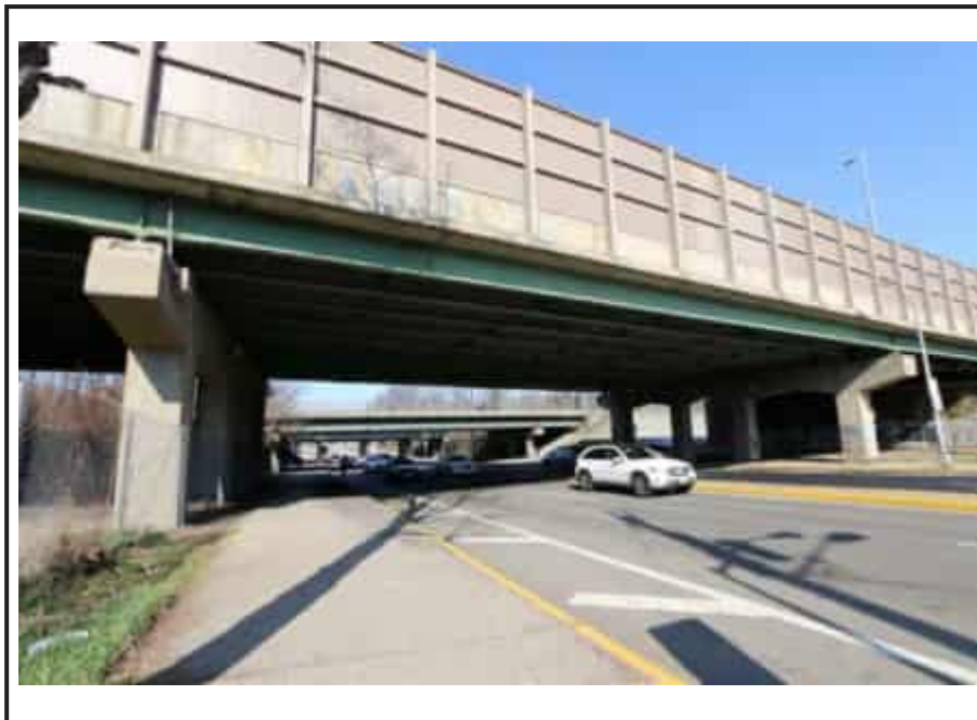
Overview, New Jersey Turnpike Newark Bay-Hudson County Extension Bridge over JFK Boulevard depicting typical piers and stringers. Note modern sound barrier.
