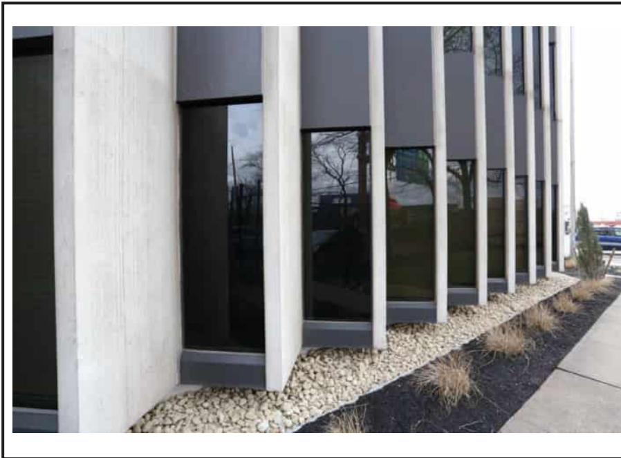
Detail view of the glass and spandrel paneling framed by the vertical precast concrete panels on the northwest elevation of the Port Authority Administration Building (Building 260).
