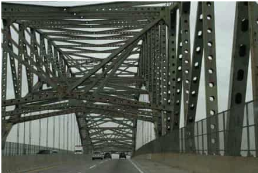
Newark Bay Bridge, east anchor arm truss span approaching the cantilevered arch truss span.
