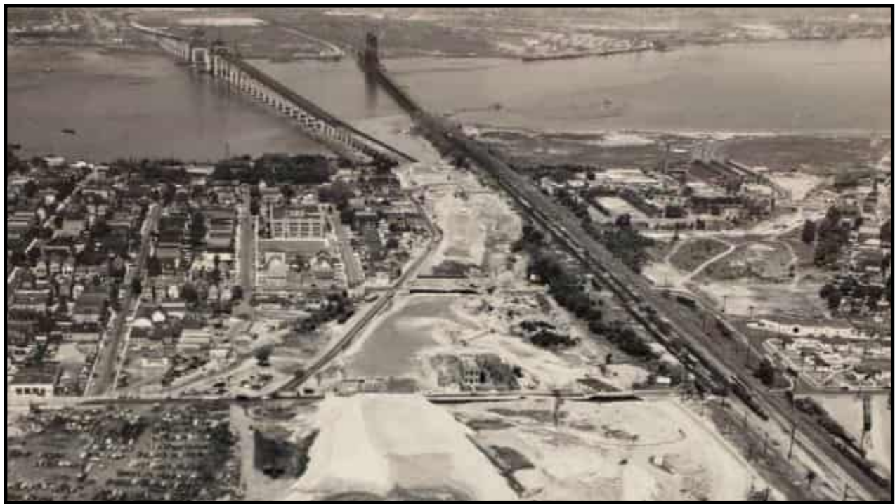
Figure 19: 1955 aerial photograph depicting early construction of the Avenue E interchange in Bayonne. The bridge's completed east and west anchor arm truss spans appear in the background, upper left (Fairchild Aerial Surveys, Inc. 1955).
