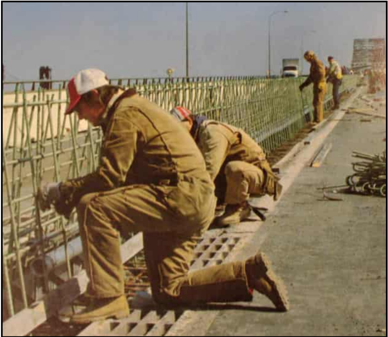
Figure 30: 1984 NJTA Annual report photograph of the demolition and replacement of the original center barrier on the Newark Bay Bridge (NJTA 1985: 5).
