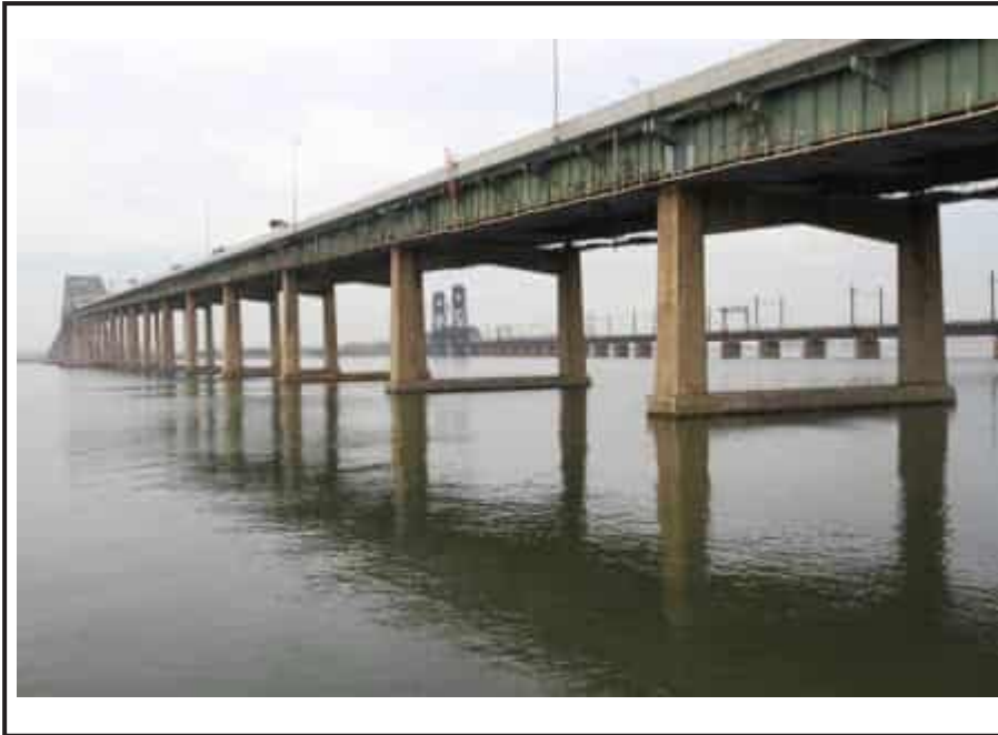
Newark Bay Bridge, overview of the south elevation and east approach depicting typical water piers and girder spans.
