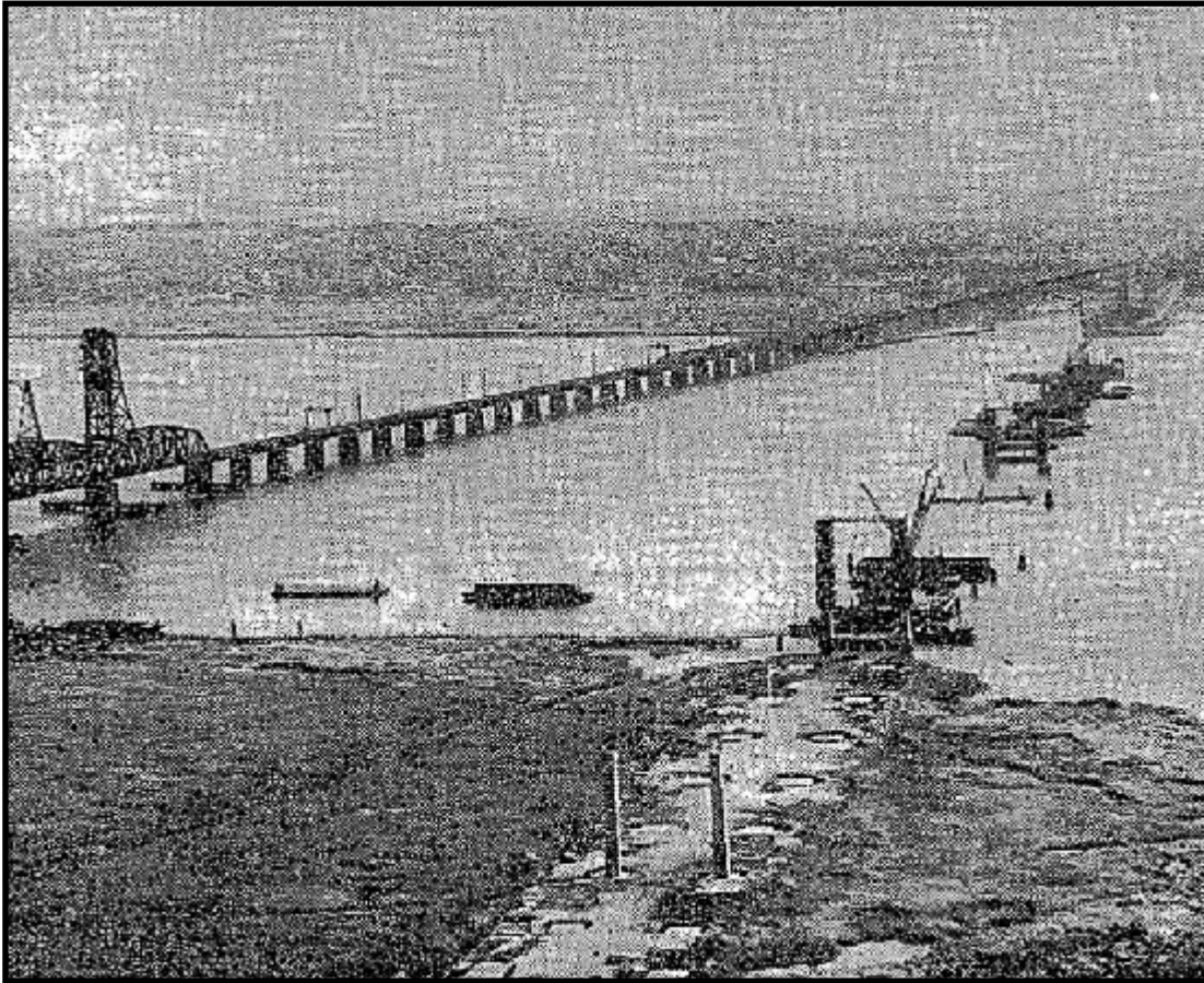
Figure 16: 1954 newspaper aerial photograph depicting the west approach fill, pier foundations, and pier construction, looking east (NYT 16 September 1954b: 31).
