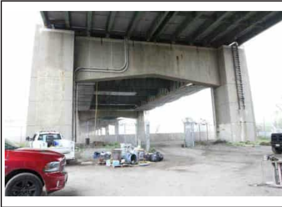
Newark Bay Bridge, depicting Pier E19 at the junction between the beam spans (steel stringers) and the girder spans on the east approach.
