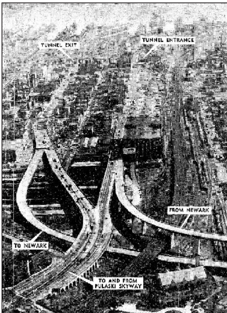
Figure 29: 1956 NJTA Annual Report photograph from the vicinity of the former Erie Railroad viaduct (foreground) depicting the completed Newark Bay-Hudson County Extension's extensive use of elevated viaducts, which contributed to the project's large expense. Clearances between piers dictated the use of girder spans or beam spans (NJTA 1957).
