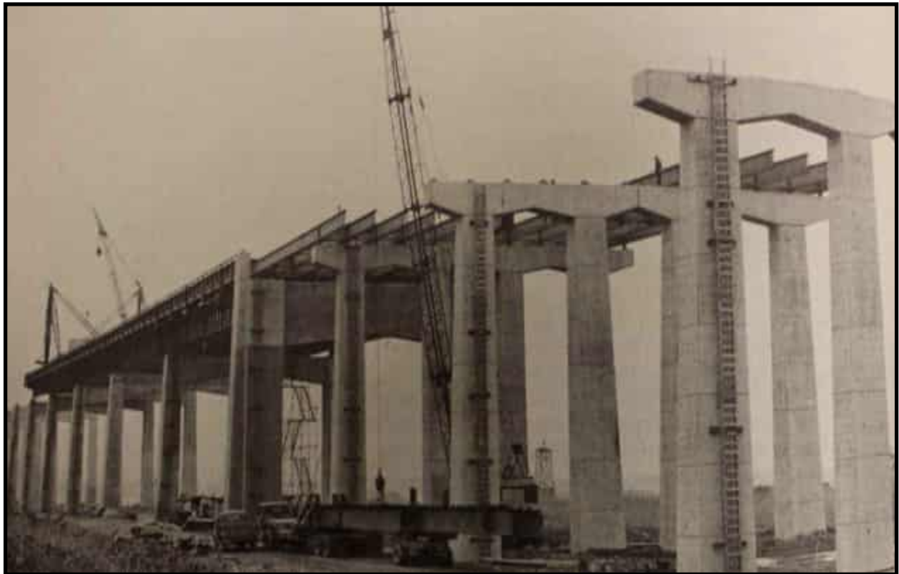
Figure 17: 1954 NJTA Annual Report photograph depicting construction of the west approach at the junction between the beam spans (foreground) and the girder spans (background) (NJTA 1955: 34).
