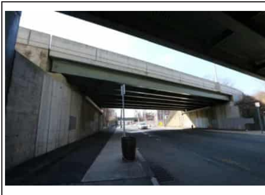
New Jersey Turnpike Newark Bay-Hudson County Extension Ramp C Bridge over Garfield Avenue. Note modern solid concrete parapet wall.
