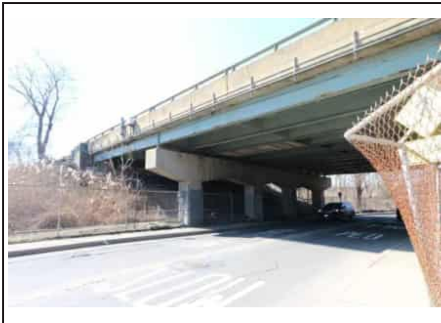
New Jersey Turnpike Newark Bay-Hudson County Extension Bridge over Linden Avenue depicting typical abutments, piers, stringer superstructure, and original pipe railing.
