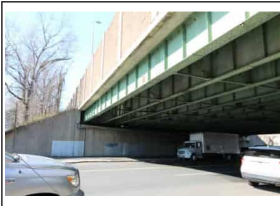
Overview, New Jersey Turnpike Newark Bay-Hudson County Extension Bridge over Avenue C depicting typical abutments and built-up girders. Note modern sound barrier.
