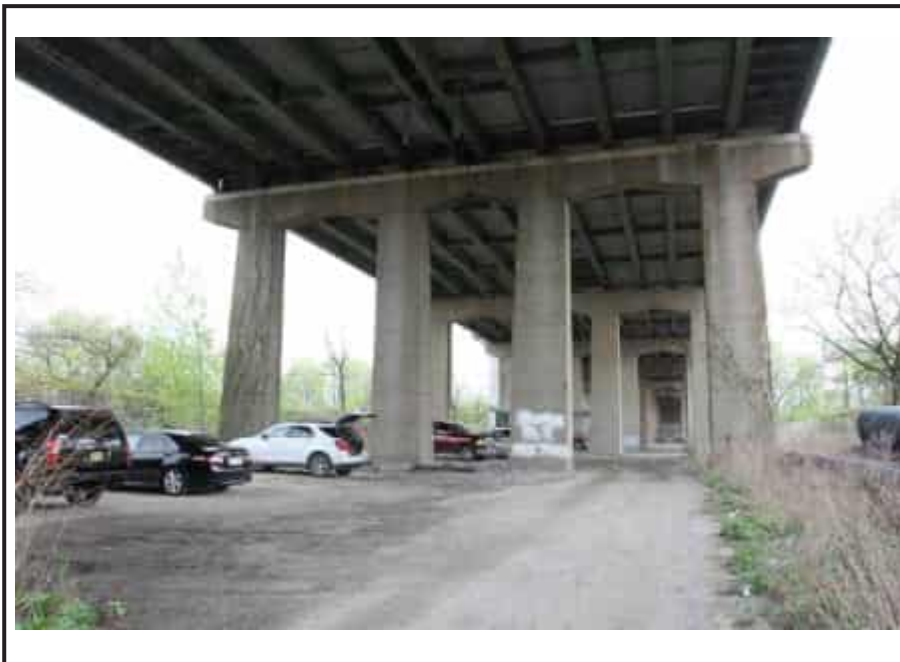
Newark Bay Bridge, depicting Pier E22 and a typical overview of the beam spans on the east approach. Note paired configuration of piers supporting eastbound and westbound lanes.
