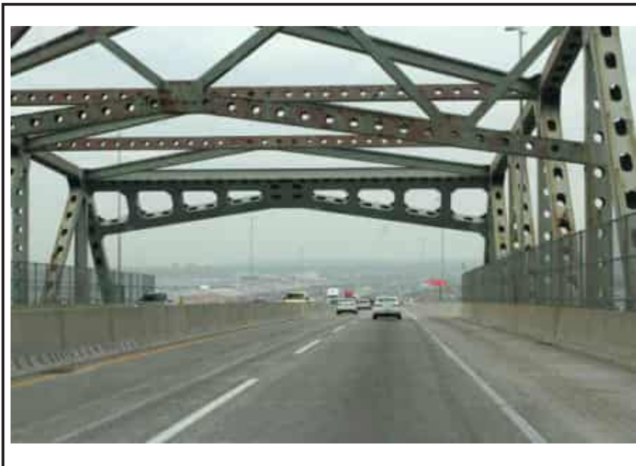
Newark Bay Bridge, west anchor arm truss span and west portal.
