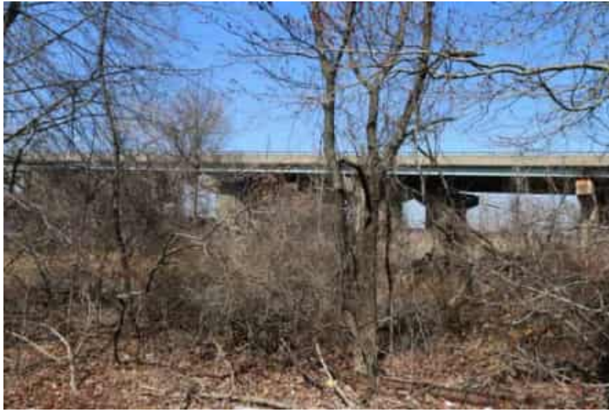
The New Jersey Turnpike Newark Bay-Hudson County Extension Bayview Viaduct depicting typical piers, stringer superstructure, and original pipe railing.
