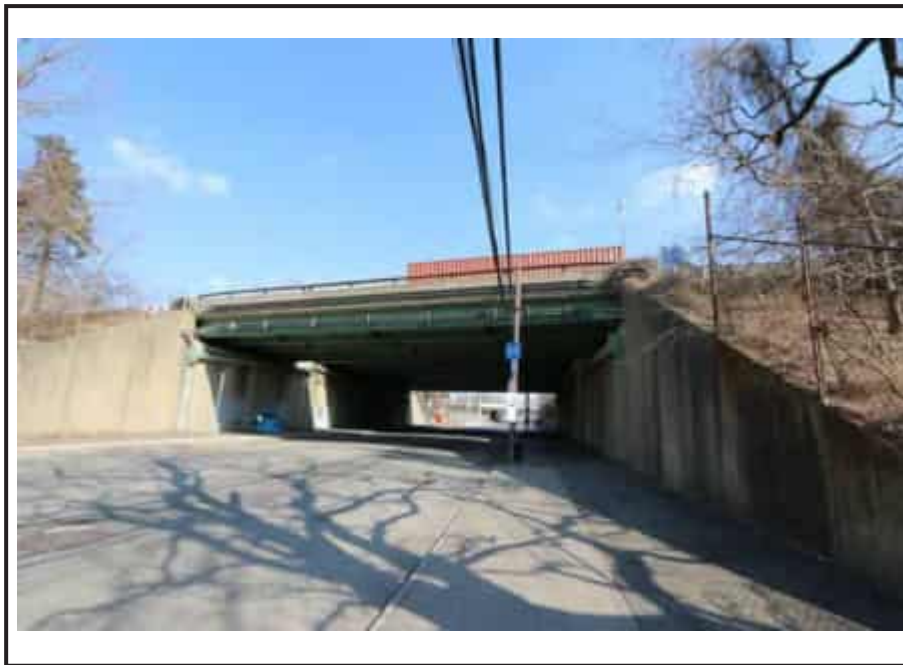
New Jersey Turnpike Newark Bay-Hudson County Extension Bridge and Ramp A over Garfield Avenue depicting typical abutments and wingwalls. Note original stormwater drains and pipe railing.
