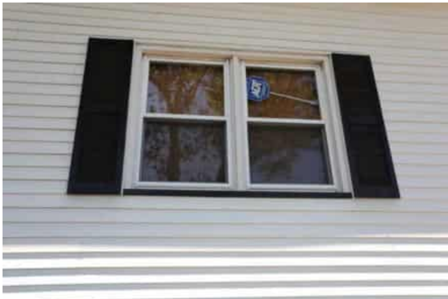
A detail view of paired, double-hung, vinyl-sash window units with inoperable shutters on the southeast elevation of 61 West 56th Street.
