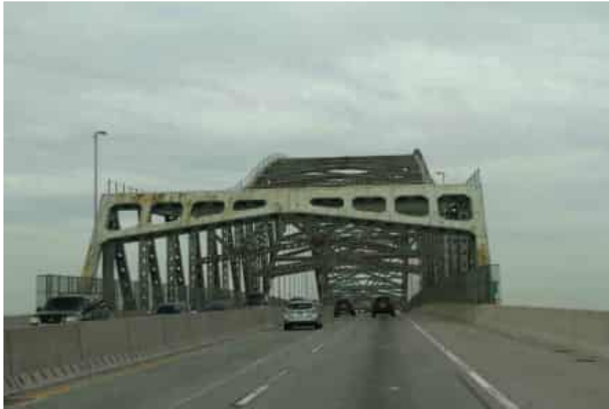
Newark Bay Bridge, east anchor arm truss span portal. Center roadway divider and outer parapets are recent replacements.
