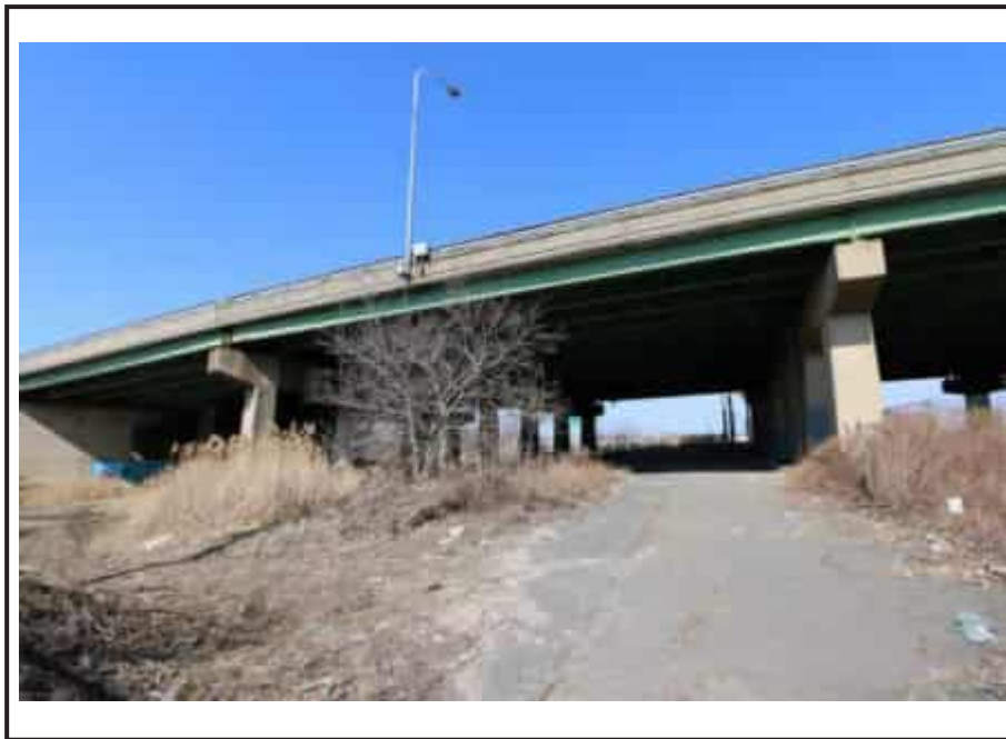
New Jersey Turnpike Newark Bay-Hudson County Extension Southeast Viaduct and Ramp D depicting typical abutments, piers, stringer superstructure, and original pipe railing.
