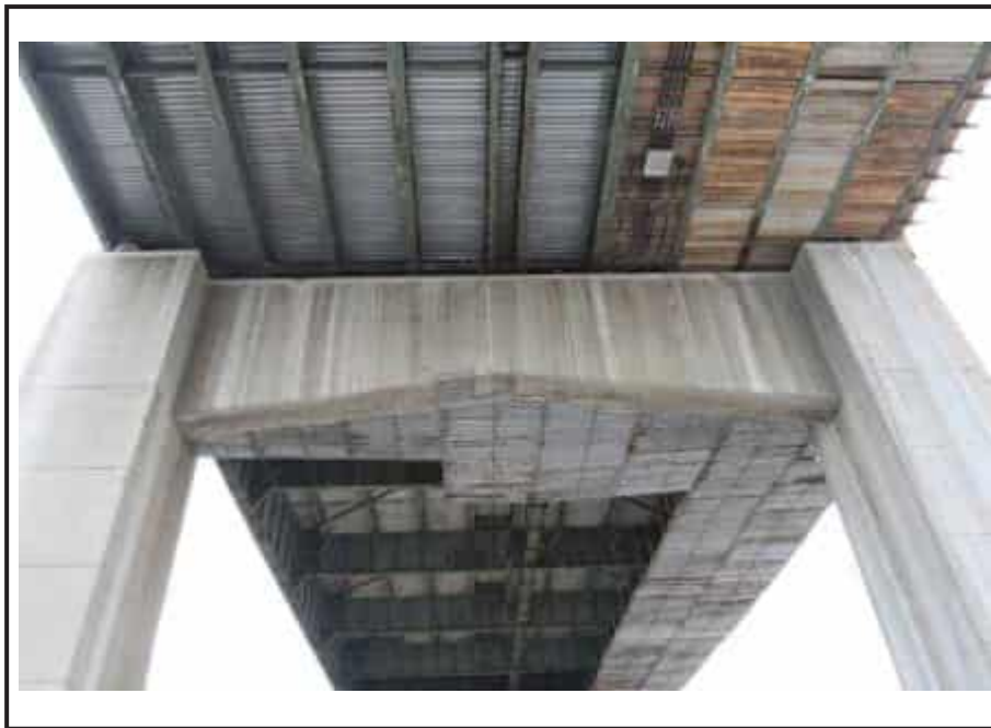
Newark Bay Bridge, depicting Pier W15 at the junction between the beam spans and girder spans of the west approach.
