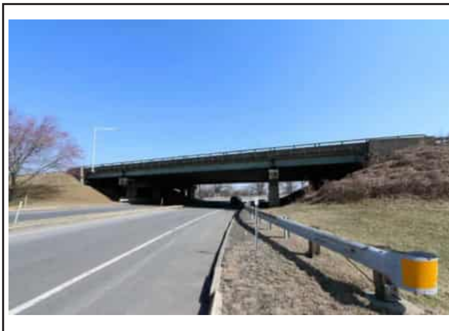
New Jersey Turnpike Newark Bay-Hudson County Extension Bridge over Ramps B and C at the Jersey City Interchange, depicting typical earthen embankments, abutments, piers, stringer superstructure, and original pipe railing.
