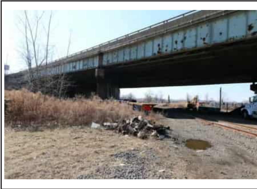
New Jersey Turnpike Newark Bay-Hudson County Extension Bridge over the former CRRNJ right of way, depicting typical solid concrete railroad crash-resistant piers, built-up girder superstructure, and original pipe railing.
