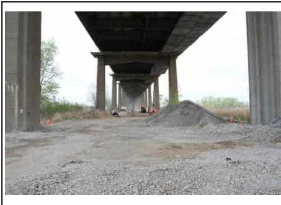
Newark Bay Bridge, depicting Pier W14 and a general overview of the single-pier substructures supporting the girder spans of the west approach.
