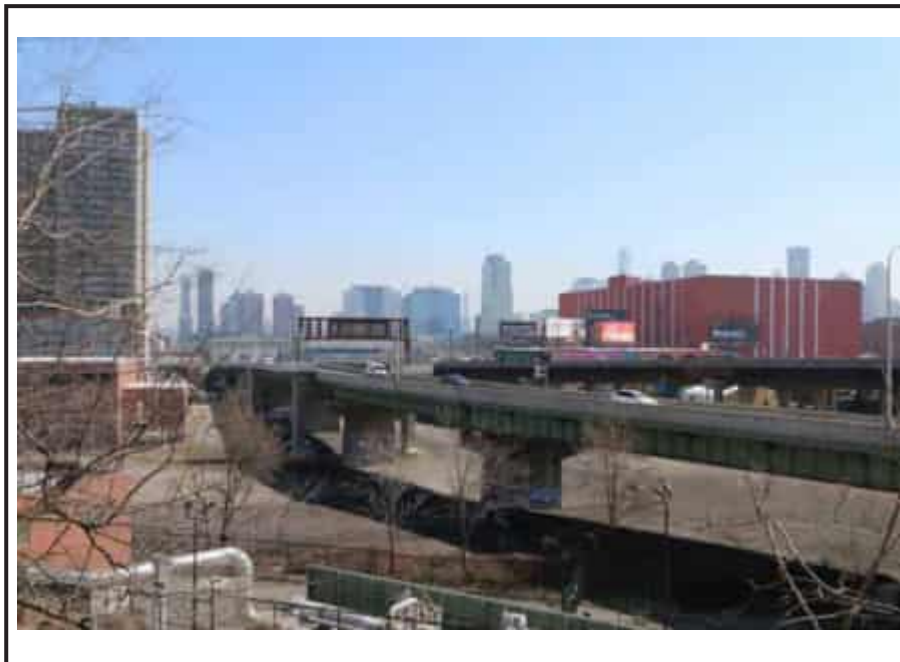
New Jersey Turnpike Newark Bay-Hudson County Extension North Terminal Ramp (westbound) over the former ERR, Conrail, PRR, and H&MRR (PATH) rights-of-way, depicting typical solid concrete railroad crash-resistant piers, built-up girder superstructure, and modern solid concrete parapet walls. Note modern overhead sign structure.
