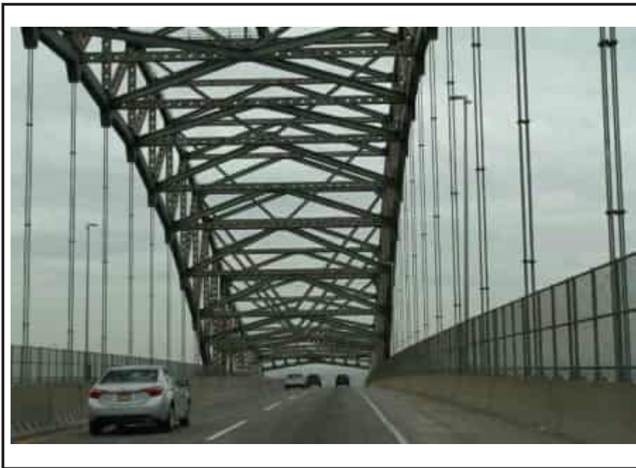
Newark Bay Bridge, central cantilevered arch truss span with suspended road deck.
