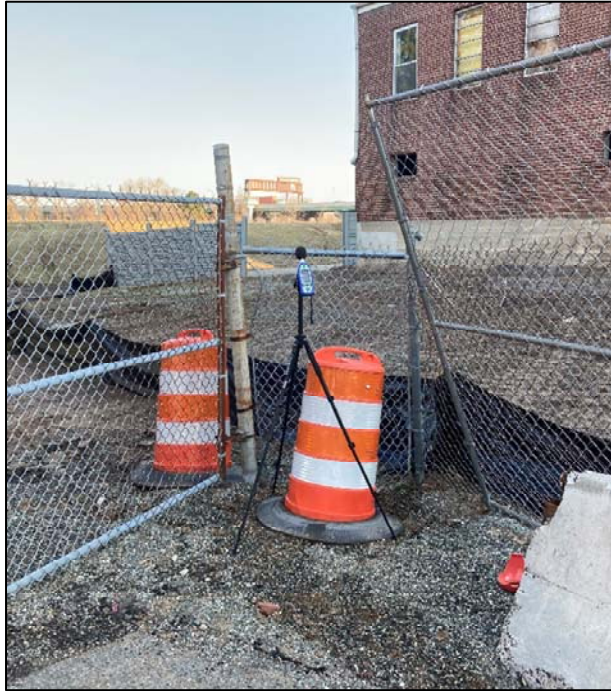
Site # 2B: 35 Sunset Drive - View Facing Northwest
