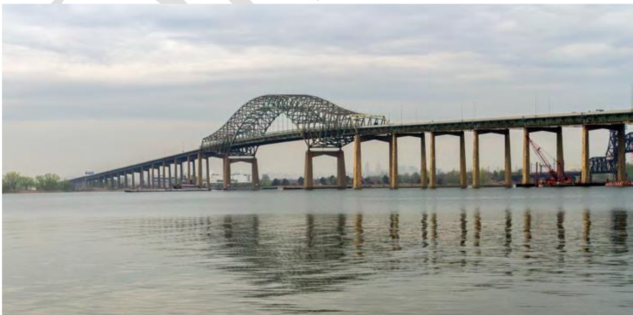
Figure 3.6-1. Existing Newark Bay Bridge
