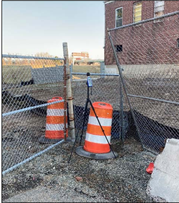
Site # 2B: 35 Sunset Drive - View Facing Northwest
