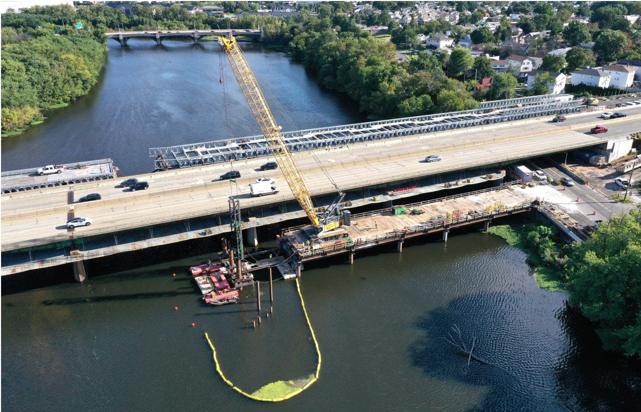
Figure 5: Superstructure Replacement and Widening of GSP Bridge Over Passaic River
