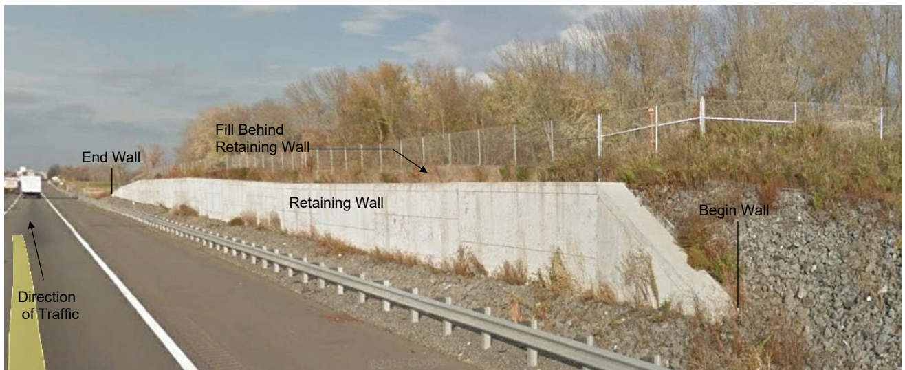
Figure 4-Standalone Retaining Wall (along Mainline shown)
