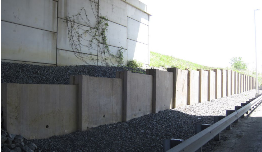
Photo 9 – Post and Panel Wall (Location – Turnpike Ramp ST, MP 53.75ST)
