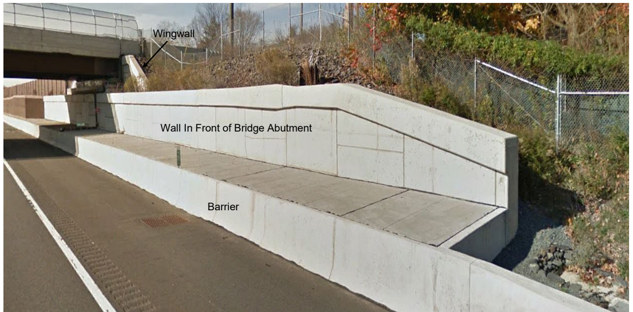
Figure 7- Wall in Front of Abutment
