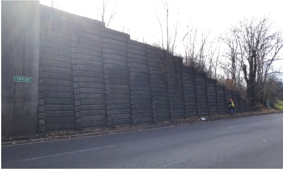
Photo 7 – Cribwall (Location – Parkway S, MP 149.4S)
