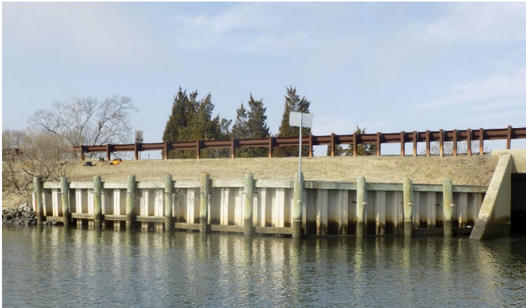
Photo 6 – Plastic Sheeting Wall (Location – Parkway N, MP 0.5N SE)
