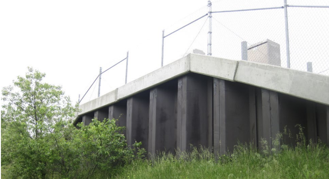
Photo 3 – Steel Sheeting Wall (Location – Parkway S, MP 31.50S)
