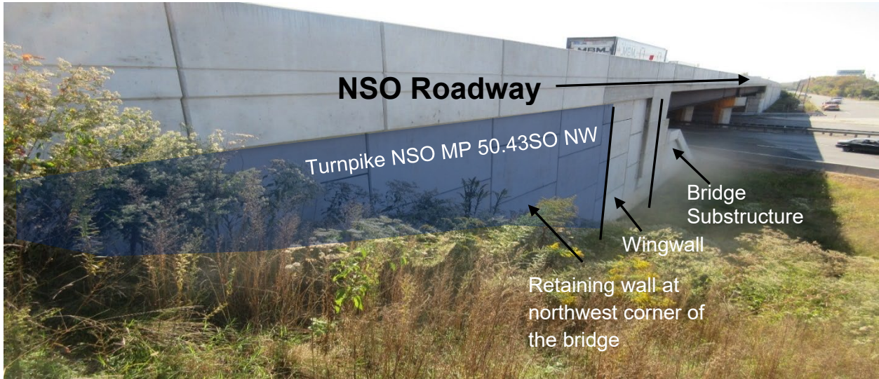
Figure 11 – Retaining Wall at Extension of Mainline Bridge (Turnpike Shown)
