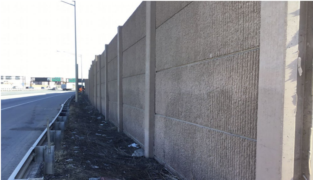
Photo 15 – Post and Panel Noise Barrier (Location – Turnpike SNO, MP 99.87NO)
