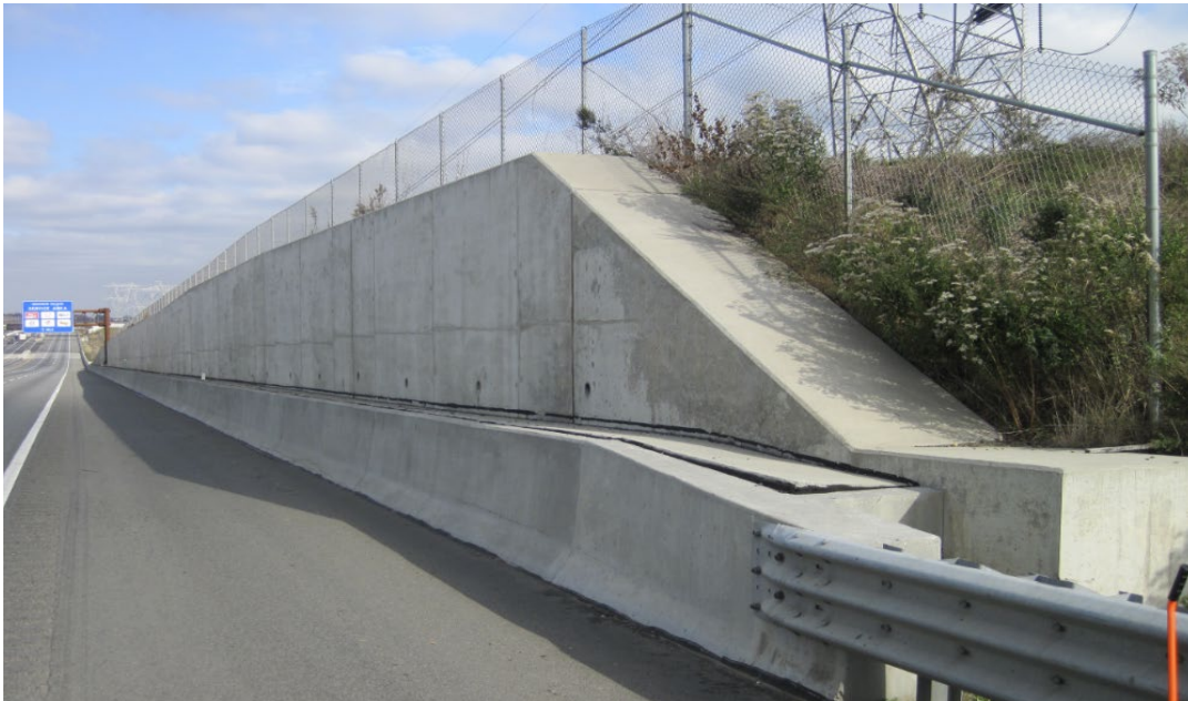
Photo 10 – Other/Combination Wall Soldier Pile Wall (Location – Turnpike SNO, MP 56.62NO)
