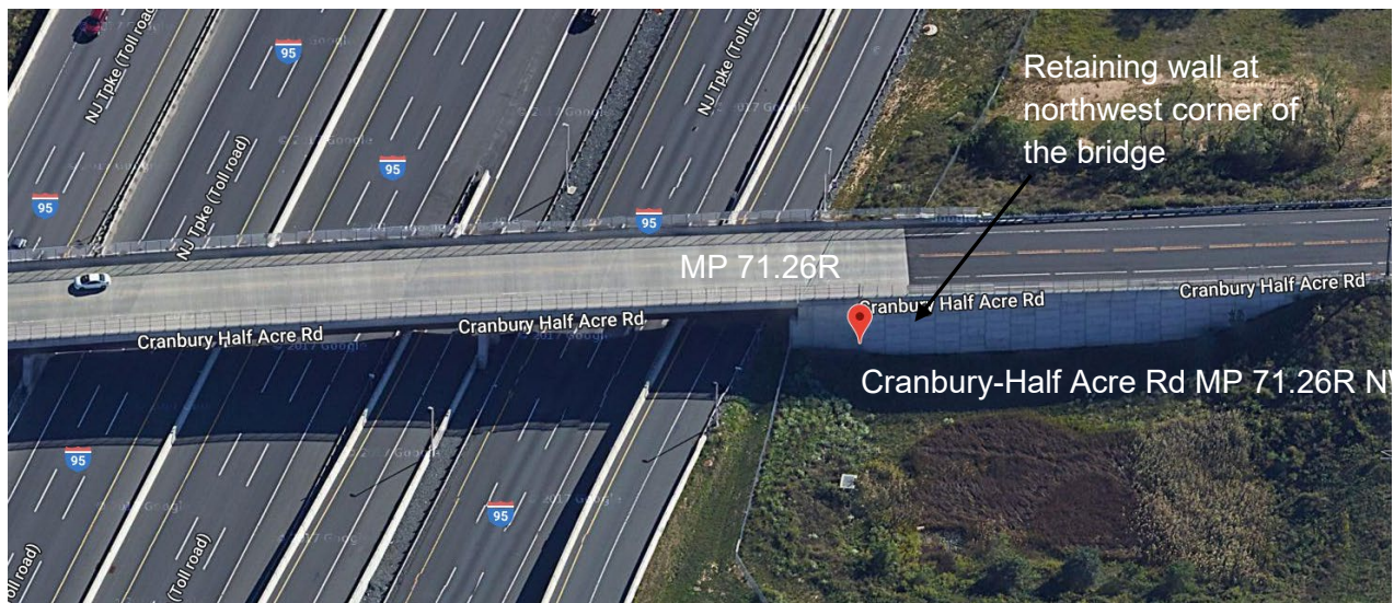
Figure 12 – Retaining Wall at Extension of Local Road Over Bridge
