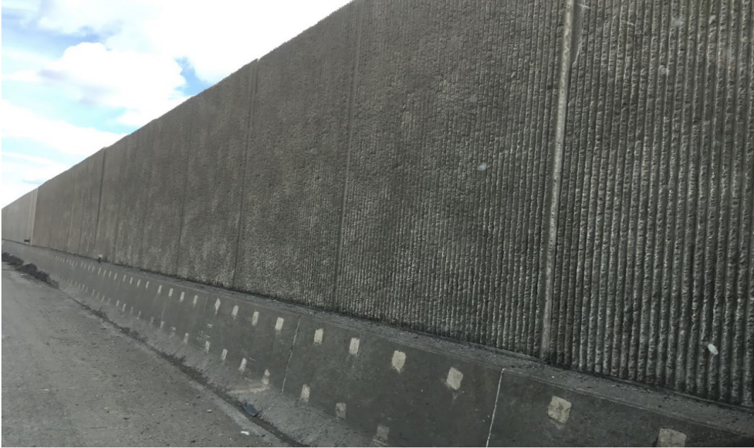
Photo 16 – Reinforced Concrete Noise Barrier (Location – Turnpike SNO, MP 100.45NO NE)
