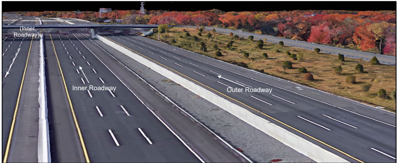
Figure 6- Median Barrier Between Outer and Inner Roadways
