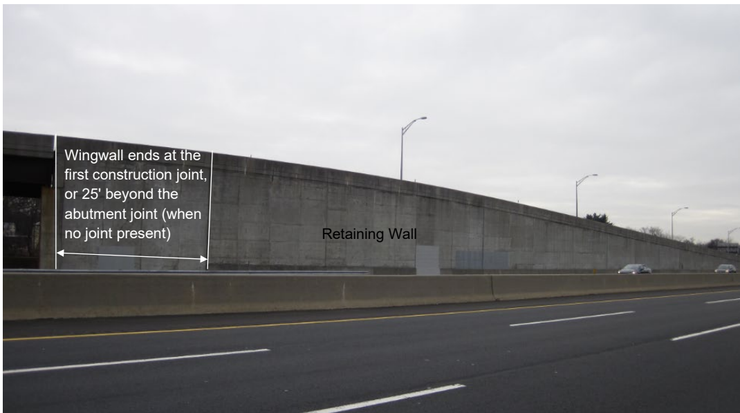
Photo 2 – Reinforced Concrete Wall (Location – Turnpike SA8N Ramp SISA, MP 78.46SW)
