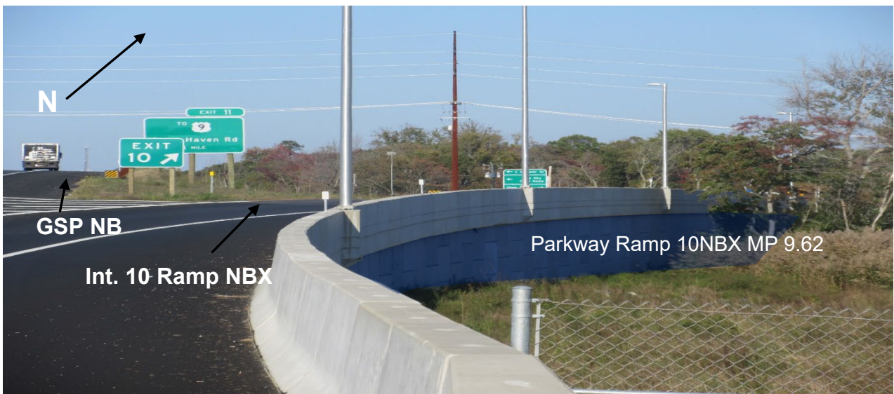
Figure 10 – Retaining Wall or Noise Barrier at Parkway Ramp
