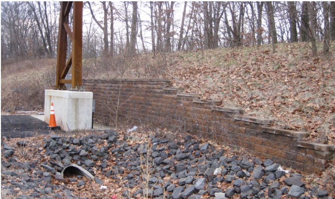
Photo 4 – Masonry Wall (Block Wall) (Location – Parkway S, MP 131.10S)
