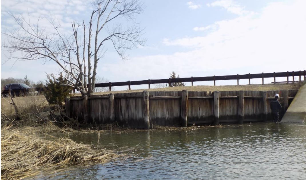
Photo 5 – Timber Sheeting Wall (Location – Parkway S, MP 2.4S NW)
