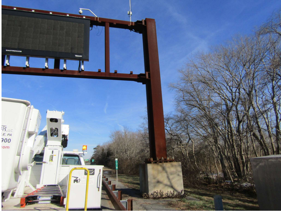
Photograph No. 5 General view of tower, looking northeast.
