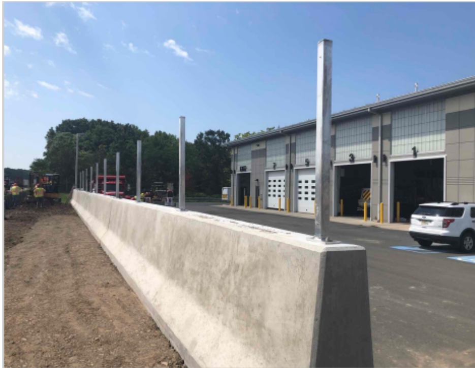
Figure 3: Installation of Barrier Fencing Express E-ZPass Lanes
