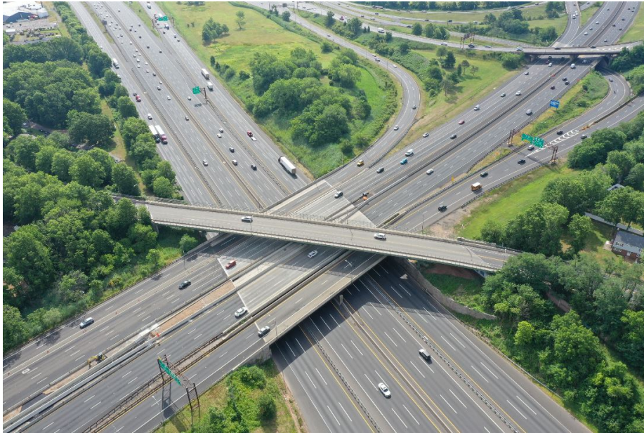
New Jersey Turnpike and Garden State Parkway Crossing in Woodbridge
