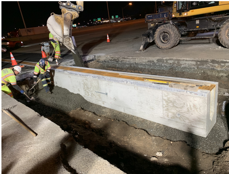
Figure 5: Installation of Trench Drain at Turnpike Interchange 14 by I-78
