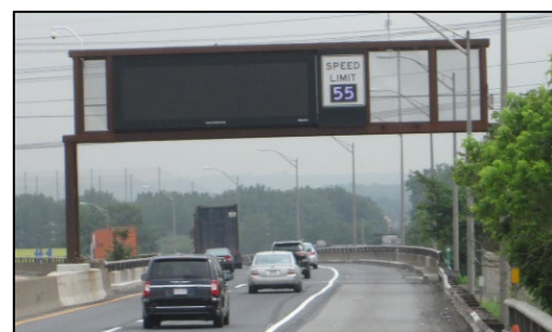
Figure 4. Fixed Electronic VMS with adjacent VSLS on overhead sign structure
