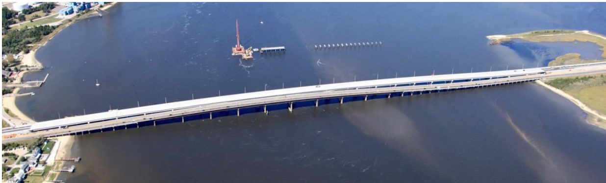
Figure 1: Great Egg Harbor Bridge Aerial View
