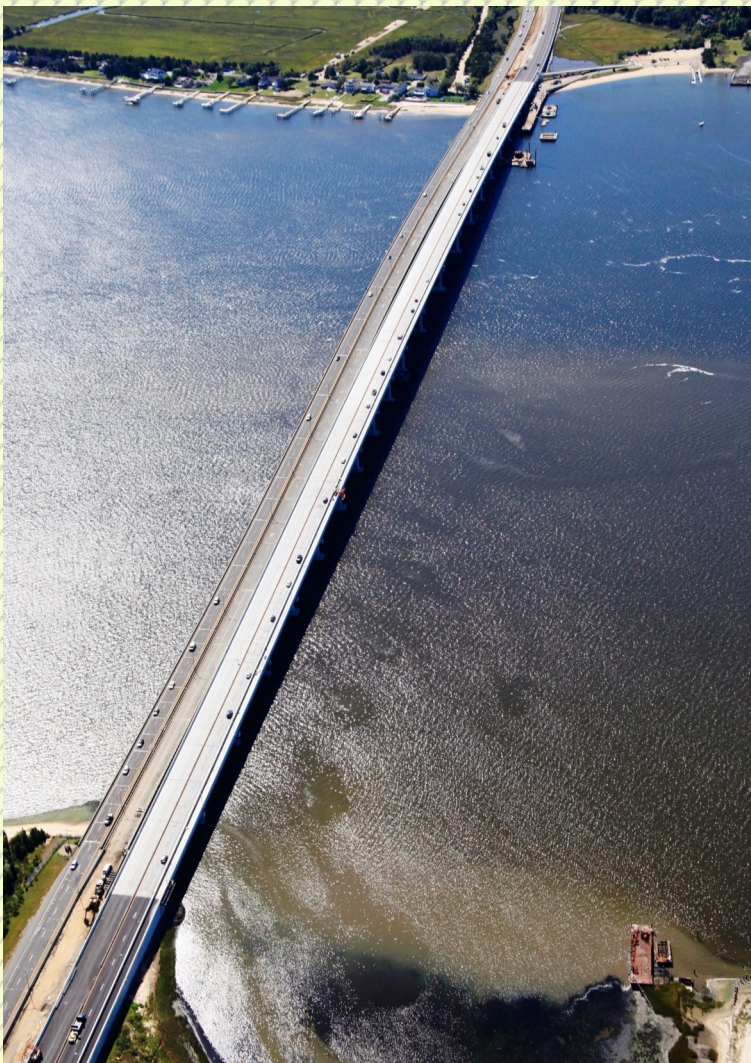
The new southbound span of the Great Egg Harbor Bridge appears on the right. A contract to rehabilitate the existing northbound span got has been underway since the fall of 2016. The old southbound span is scheduled to be demolished.
