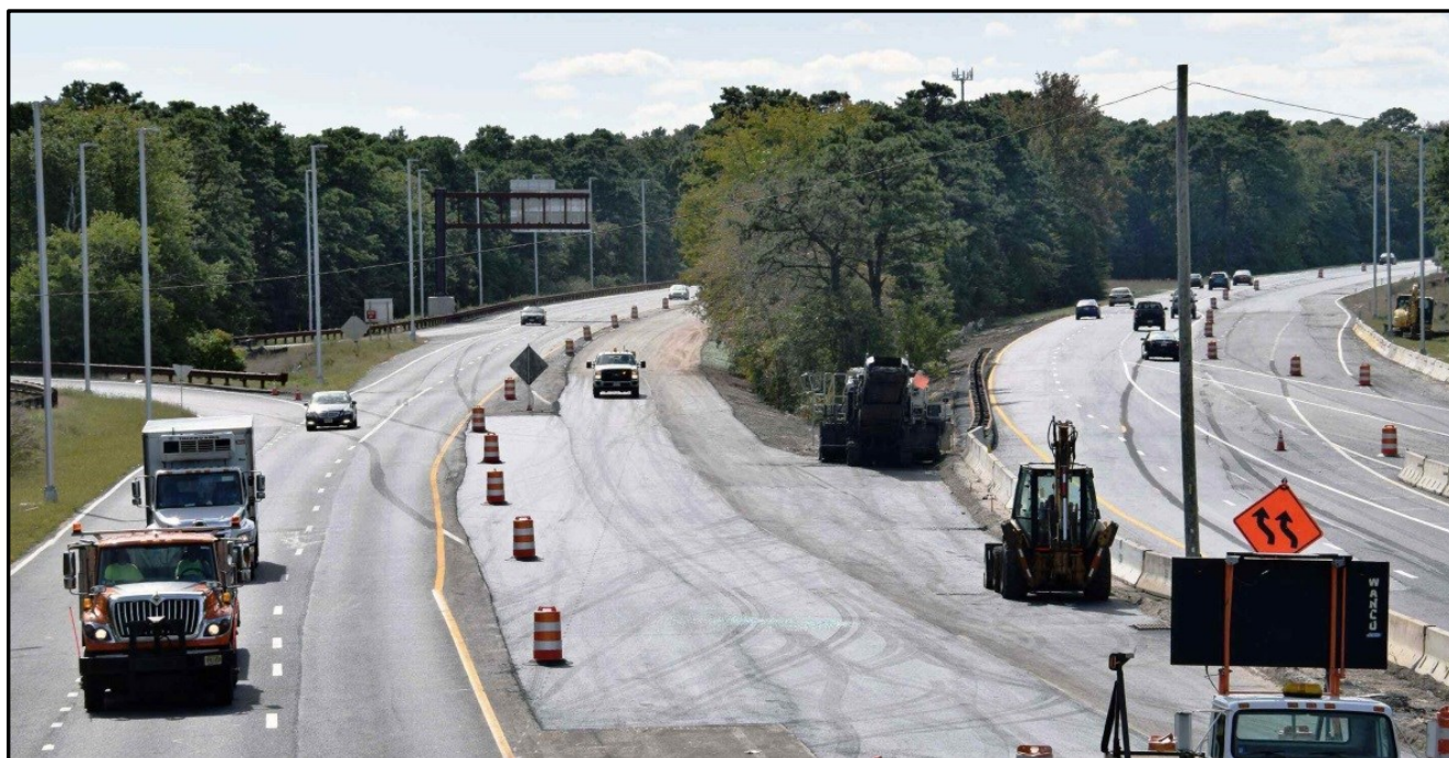
Work on phase 3 of the Garden State Parkway widening will continue through 2017. The $590 million project is adding a travel lane in each direction between mileposts 35 and 80. The first two phases are already open to traffic. This view of the progress is looking south at around milepost 36.
