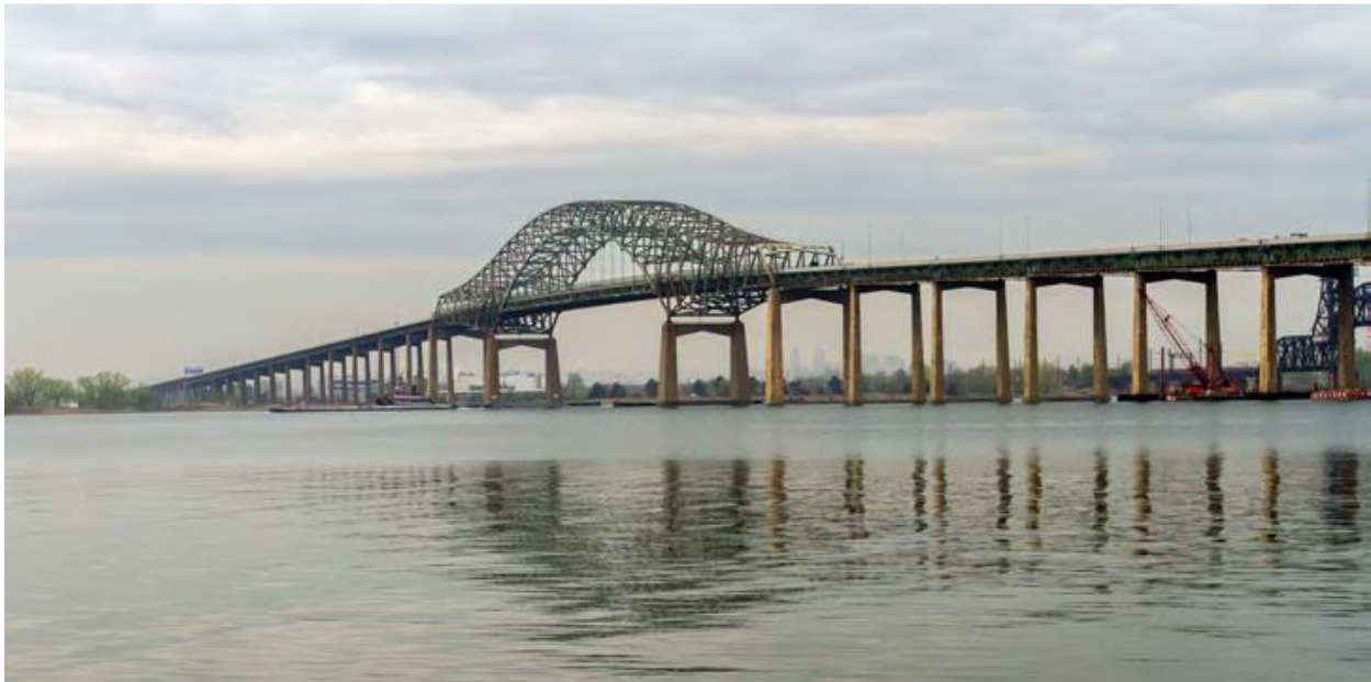
Figure 3.6-1. Existing Newark Bay Bridge
