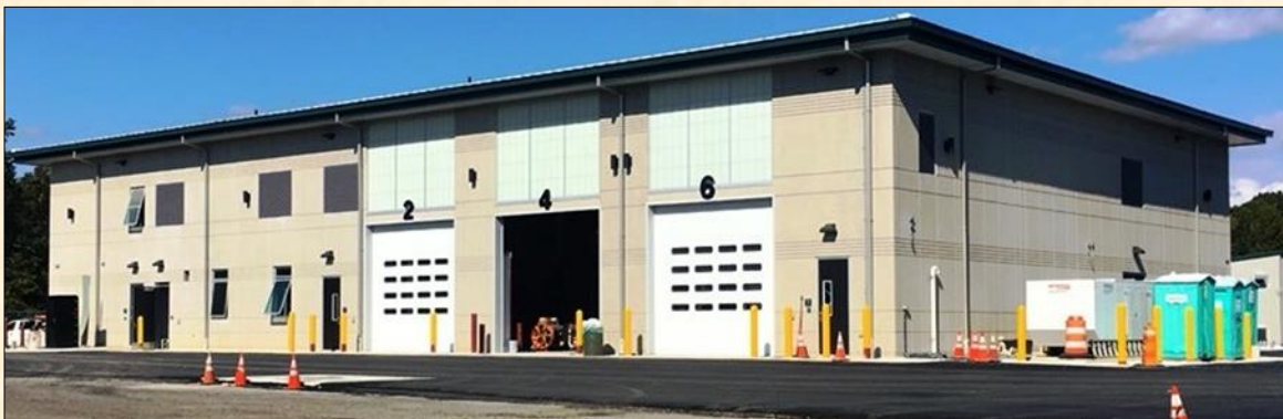
The new facility at the Swainton Maintenance Yard (Maintenance District 1) on the Garden State
