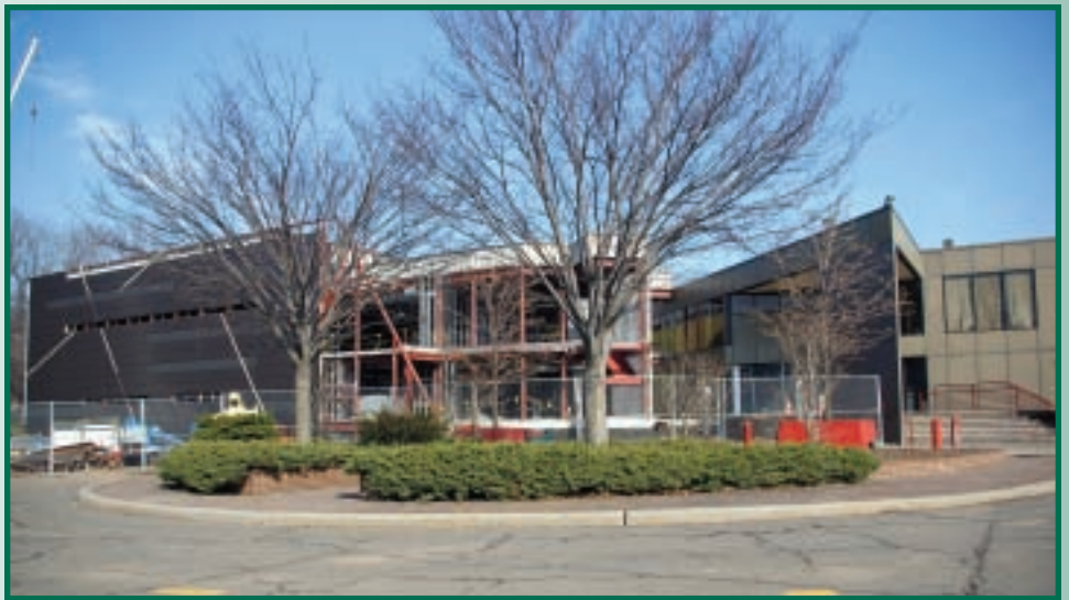
Traffic Management Center (TMC) under construction
