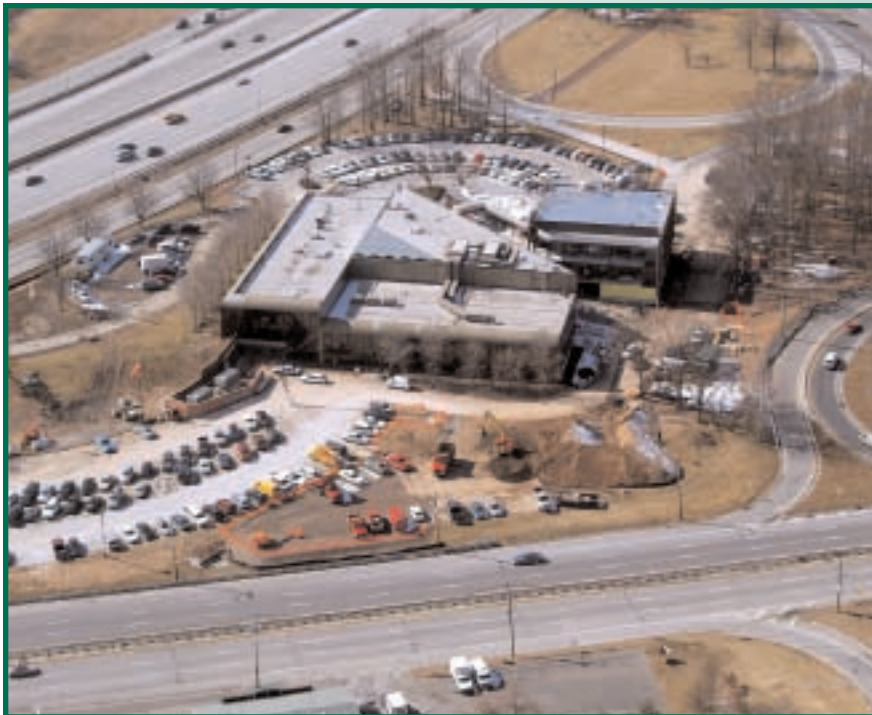
Overhead view of TMC under construction
