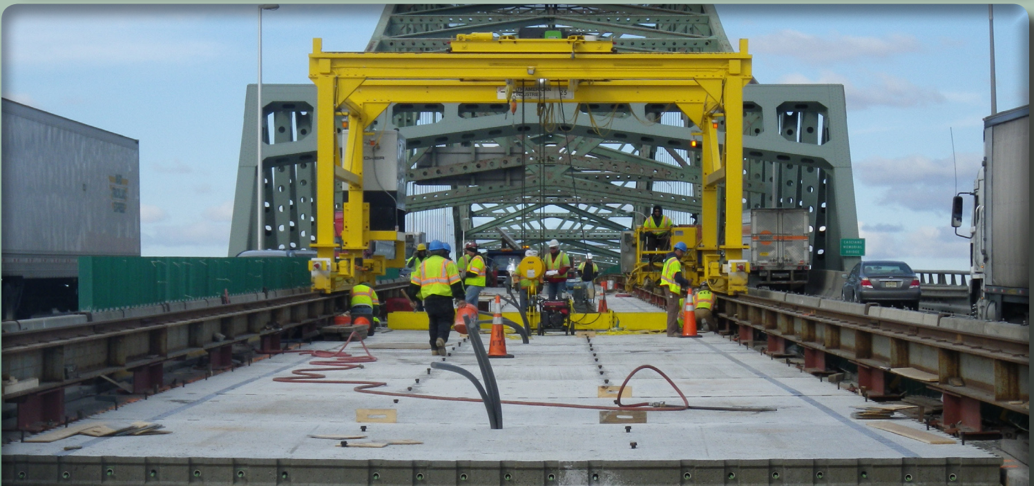
System Preservation: Replacing the deck of the Turnpike's Vincent R. Casciano Memorial Bridge in Essex and Hudson Counties
