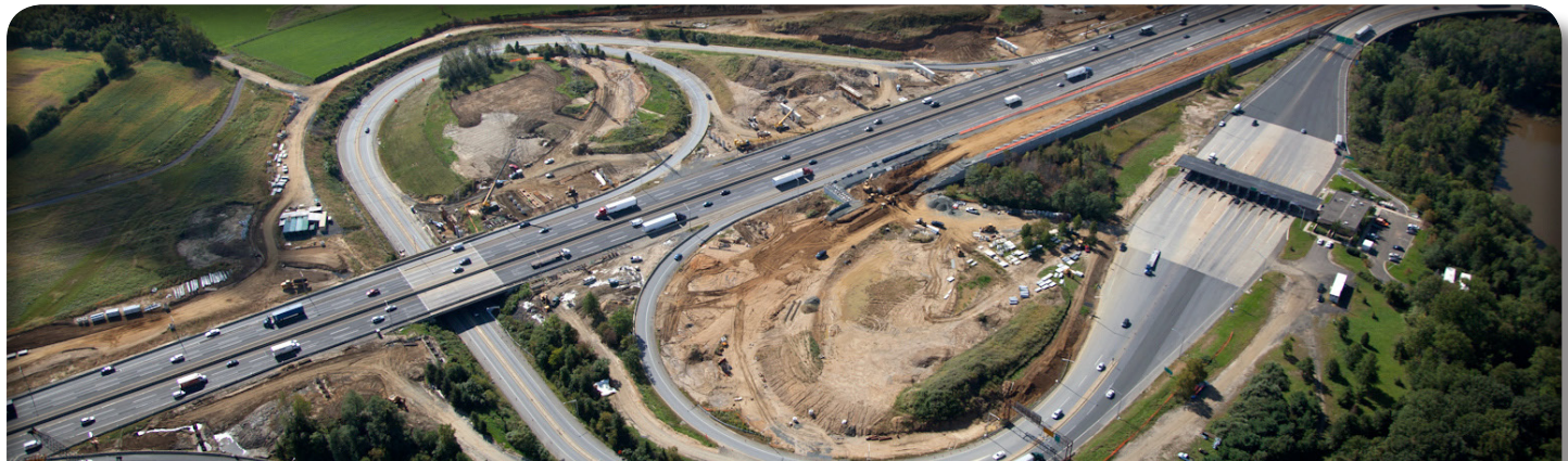
Turnpike Widening - Connections at Interchange 7
