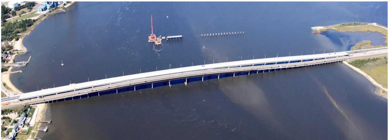
Figure 1: Great Egg Harbor Bridge Aerial View
